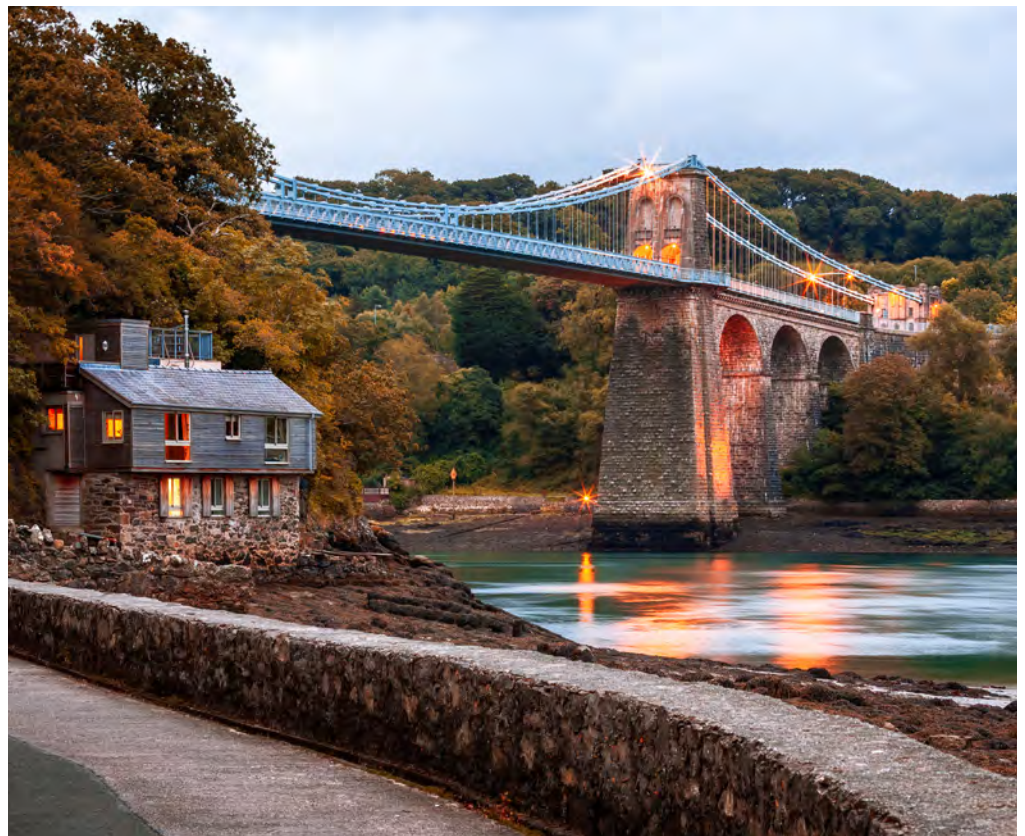
Menai Suspension Bridge, Anglesey, Wales
